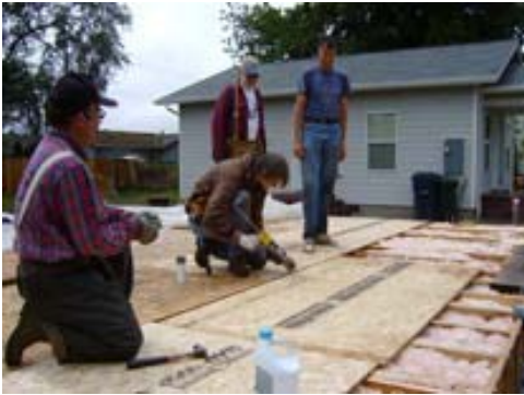
Meyer Park project, 49th and Main St., Springfield (Habitat for Humanity)
